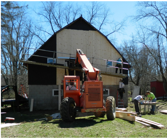
Shrock Construction covered the old horizontal siding with new vertical siding, then affixed a new door to the hay mow and gave the whole thing several coats of paint.
