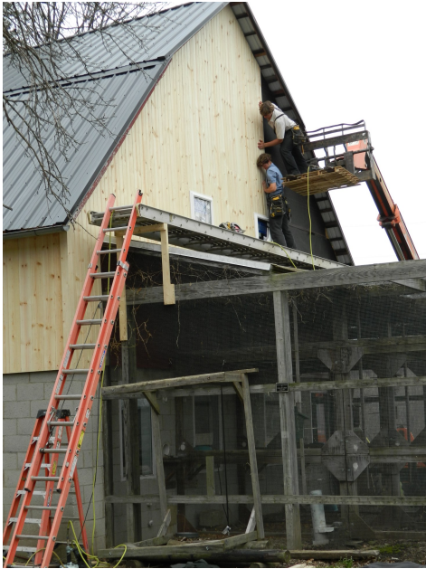
Shrock Construction covered the old horizontal siding with new vertical siding, then affixed a new door to the hay mow and gave the whole thing several coats of paint.
