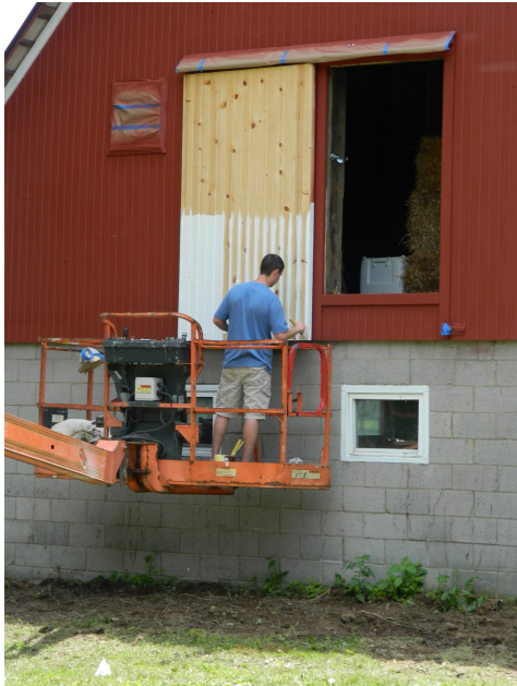
Shrock Construction covered the old horizontal siding with new vertical siding, then affixed a new door to the hay mow and gave the whole thing several coats of paint.
